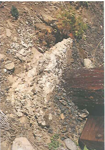
Figure 1-21: Exposed concrete base, camp end abutment downstream ballast wall pile.
