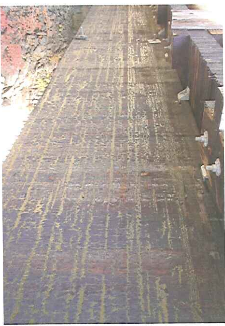
Figure 1-14: Upstream exterior girder.
