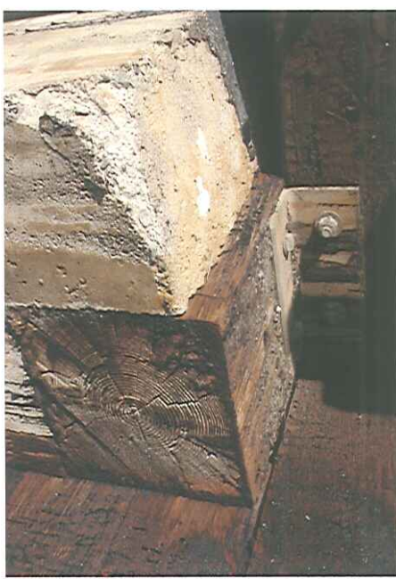
Figure 1-20: Camp end abutment timber sill.
