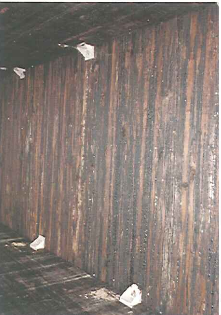
Figure 1-9: Typical condition underside of the transversely laminated structural deck.
