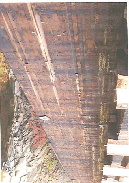
Figure 1-15: Downstream exterior girder.
