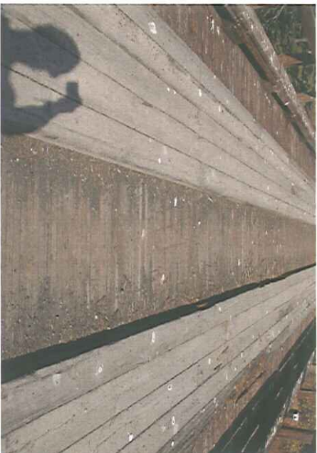
Figure 1-7: General deck condition.
